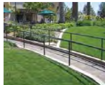
2 Concrete Ramp with Railing
