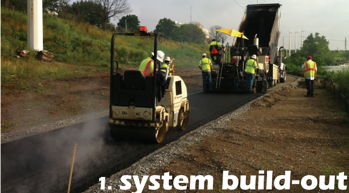
New Trail Construction along White River Greenway.
