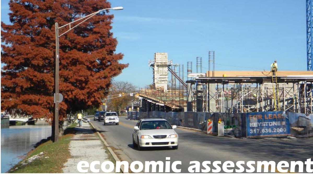
Construction activity signals new developed adjacent to the Canal Towpath.
