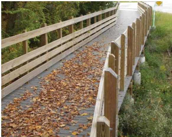
Use of boardwalks through sensitive areas.
