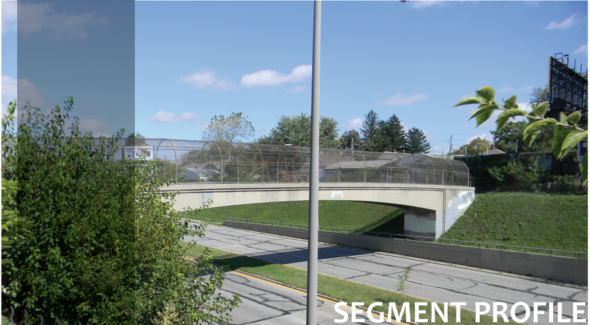
Interurban greenway corridor along Madison Avenue.
