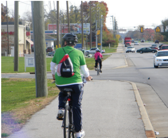
56th Street Sidewalk in Pike Township.
