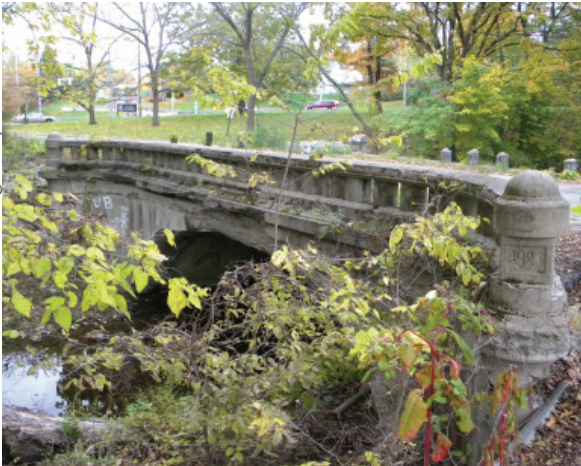
Historic Nowland Avenue bridge in Spades Park.
