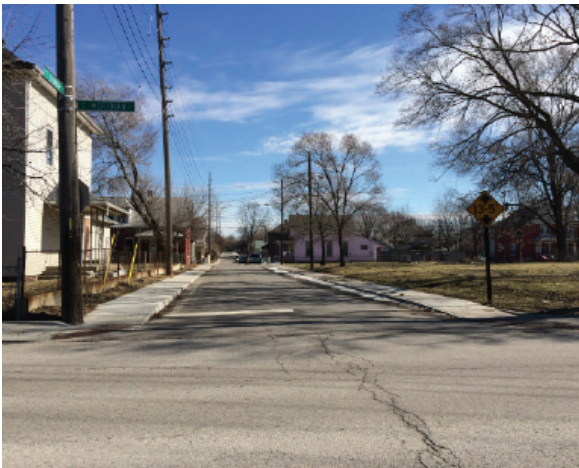
Interurban route- Orange Street bicycle boulevard.
