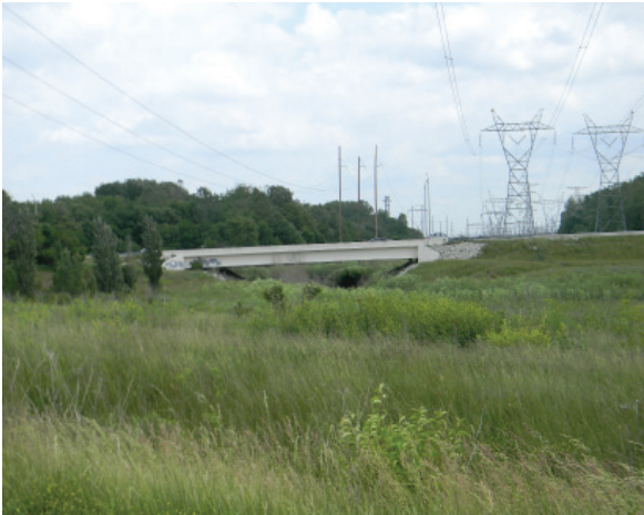
Overhead utility easement along White Lick Creek.
