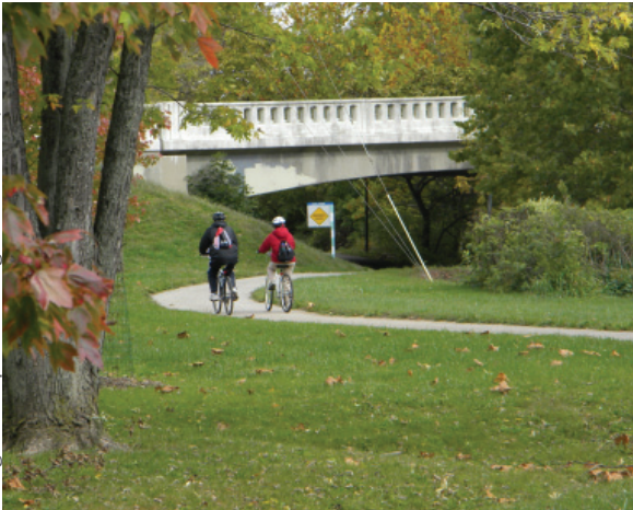
Bridge underpasses along Fall Creek at 46th Street.
