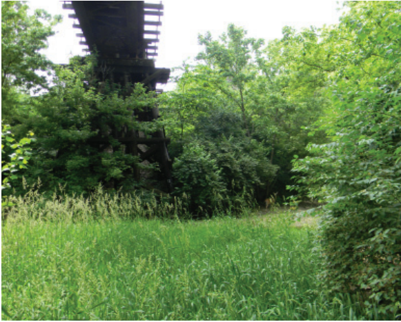
Existing railroad bridge along White Lick Creek.
